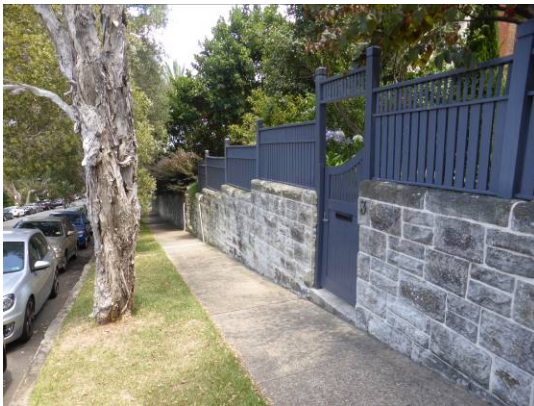
Stone wall and replica fence
