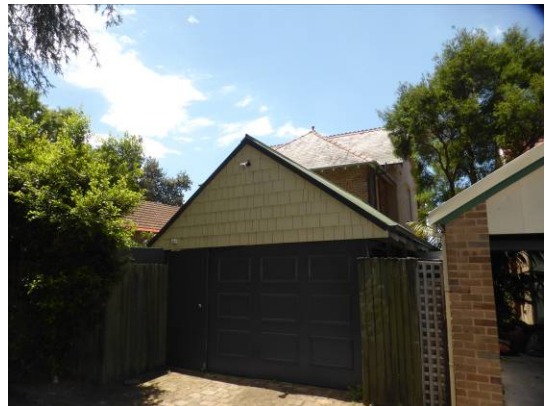
Carport to rear lane
