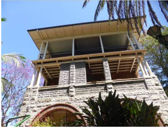
Extensive concrete block walls to facade
