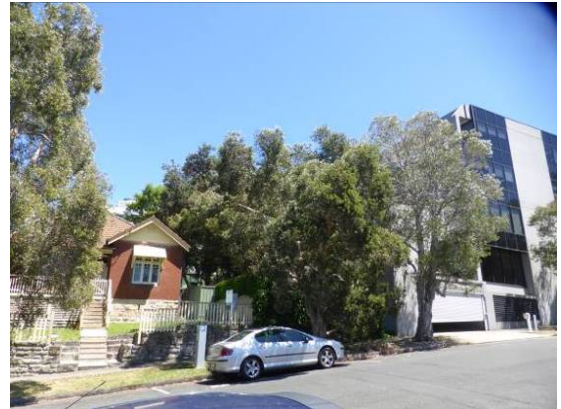
1 Park Road at rear of commercial buildings on Pacific Highway
