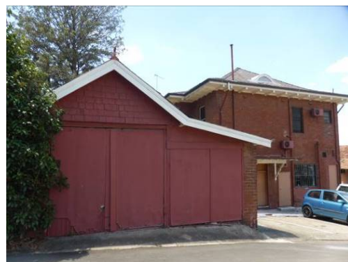
Slate roofed garage, rear of No 7
